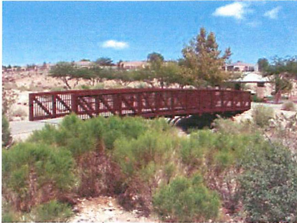
Typical steel trail bridge over a natural seasonal drainage channel
