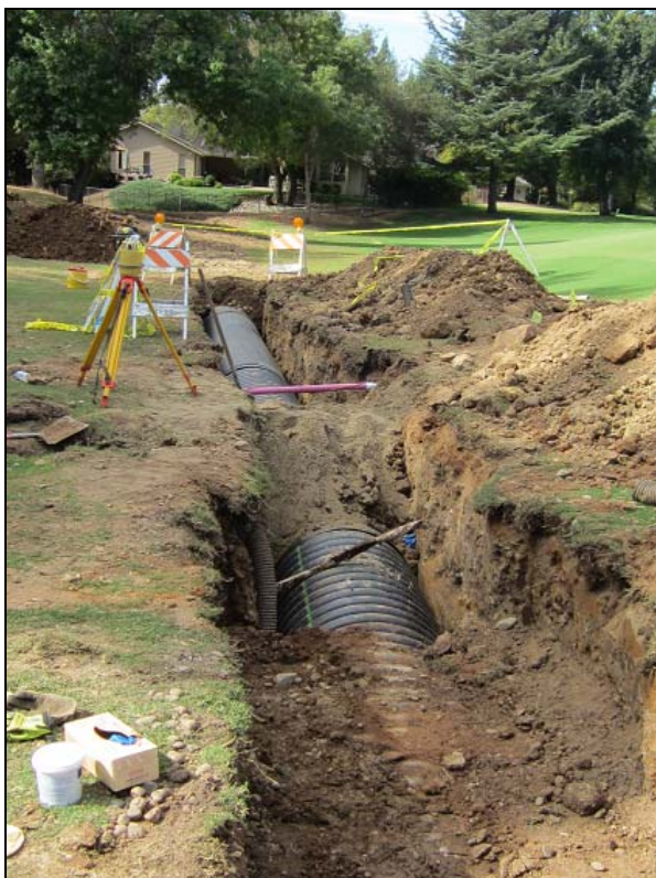
Installation of new pipe with RMCC irrigation lines running across the top of it.
