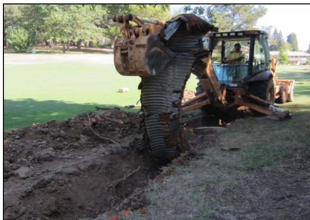
Removing the old pipe with bottom missing.
