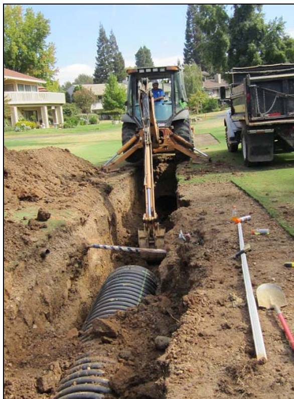
Installation of new pipe with RMCC irrigation lines running across the top of it.
