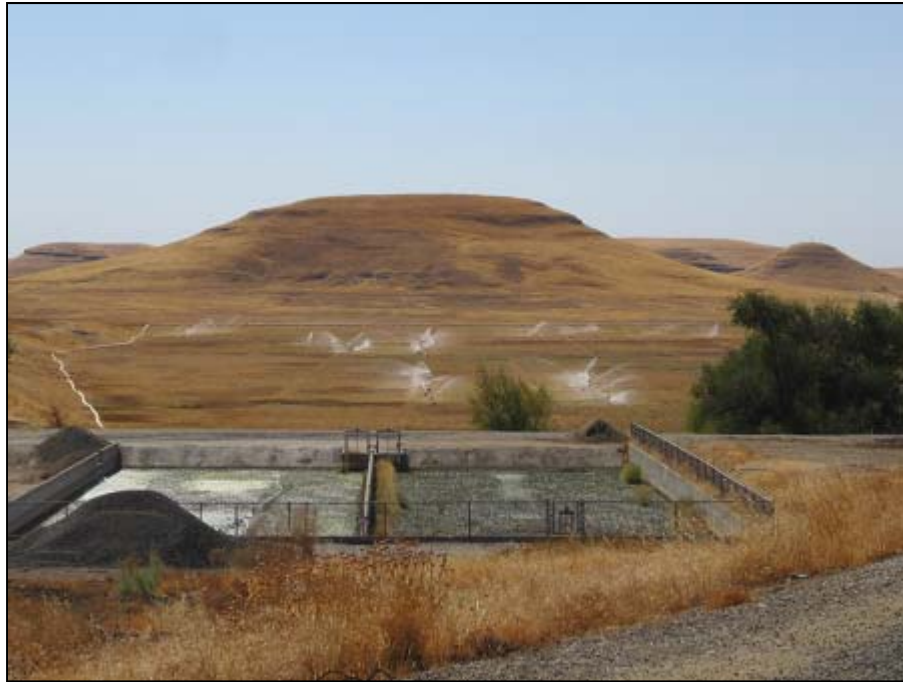
Reclaimed water irrigation at VanVleck Ranch; wastewater solids drying beds in foreground
