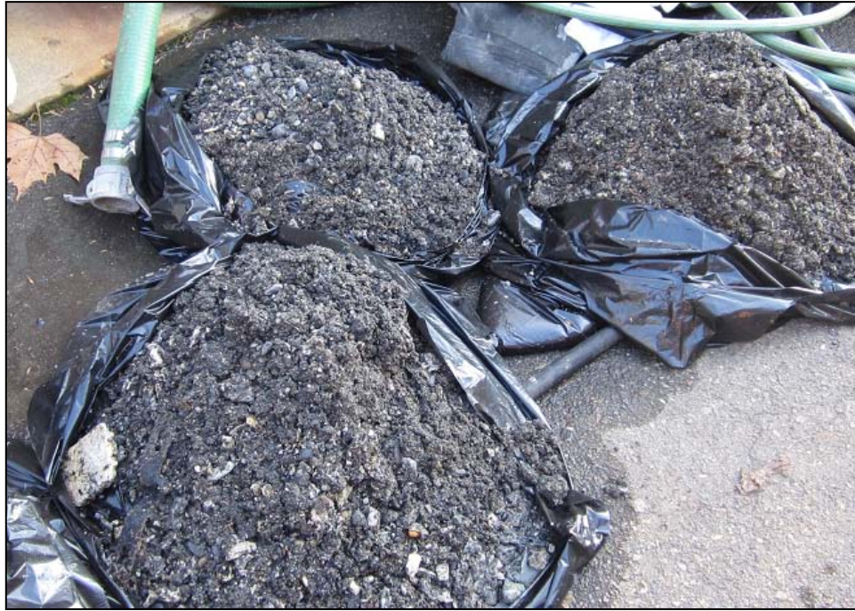
Some of the grit and debris removed from MLN wet wells.
