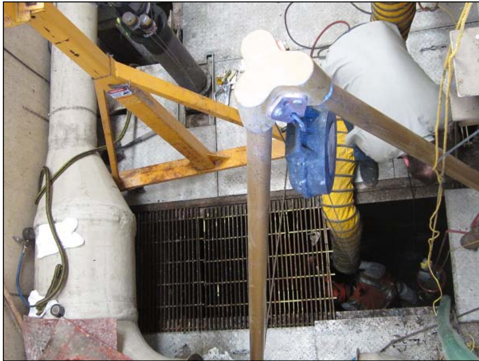
Inspector conducting inspection down in wet well #2 at MLN.
