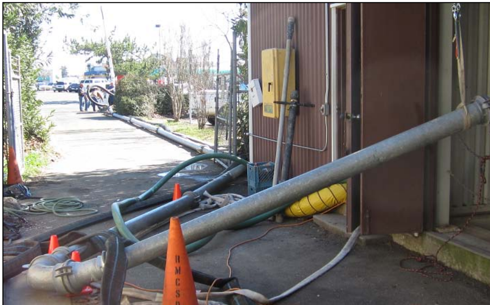
Temporary bypass piping set up by District staff.
