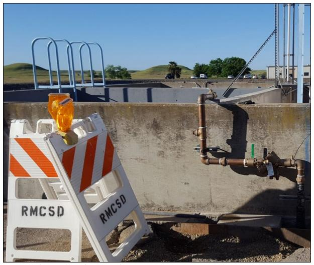
Installation of a water fill line for dilution of new chemical tanks
