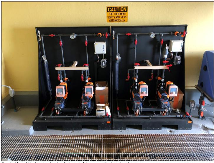
Chemical feed skids placed in chemical feed room of Wastewater Reclamation plant
