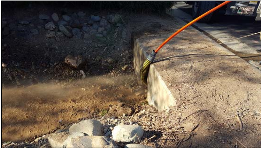
Cleaning rocks and debris out of culvert pipe at Rio Blanco
