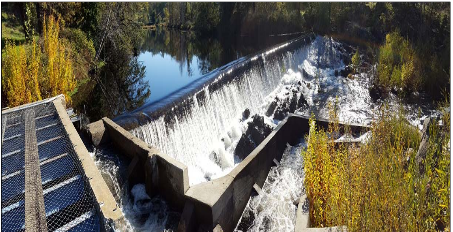
Photo of Granlees Dam with Cosumnes River flow at 232 cubic feet per second.
