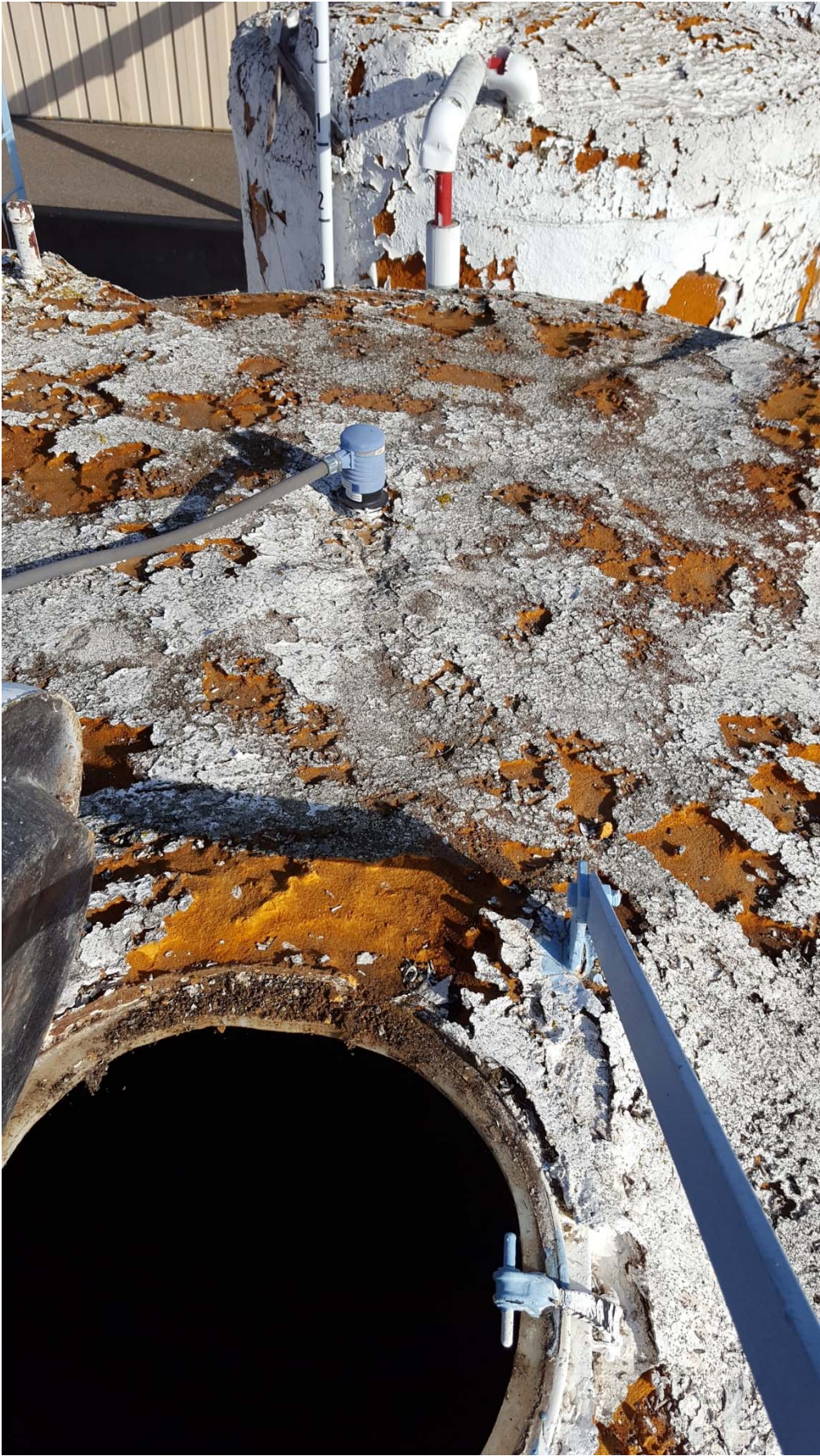
View of top of existing caustic tank with hatch open
