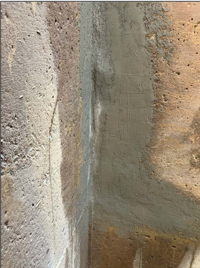
Repair made to CIA diversion box, view from inside
