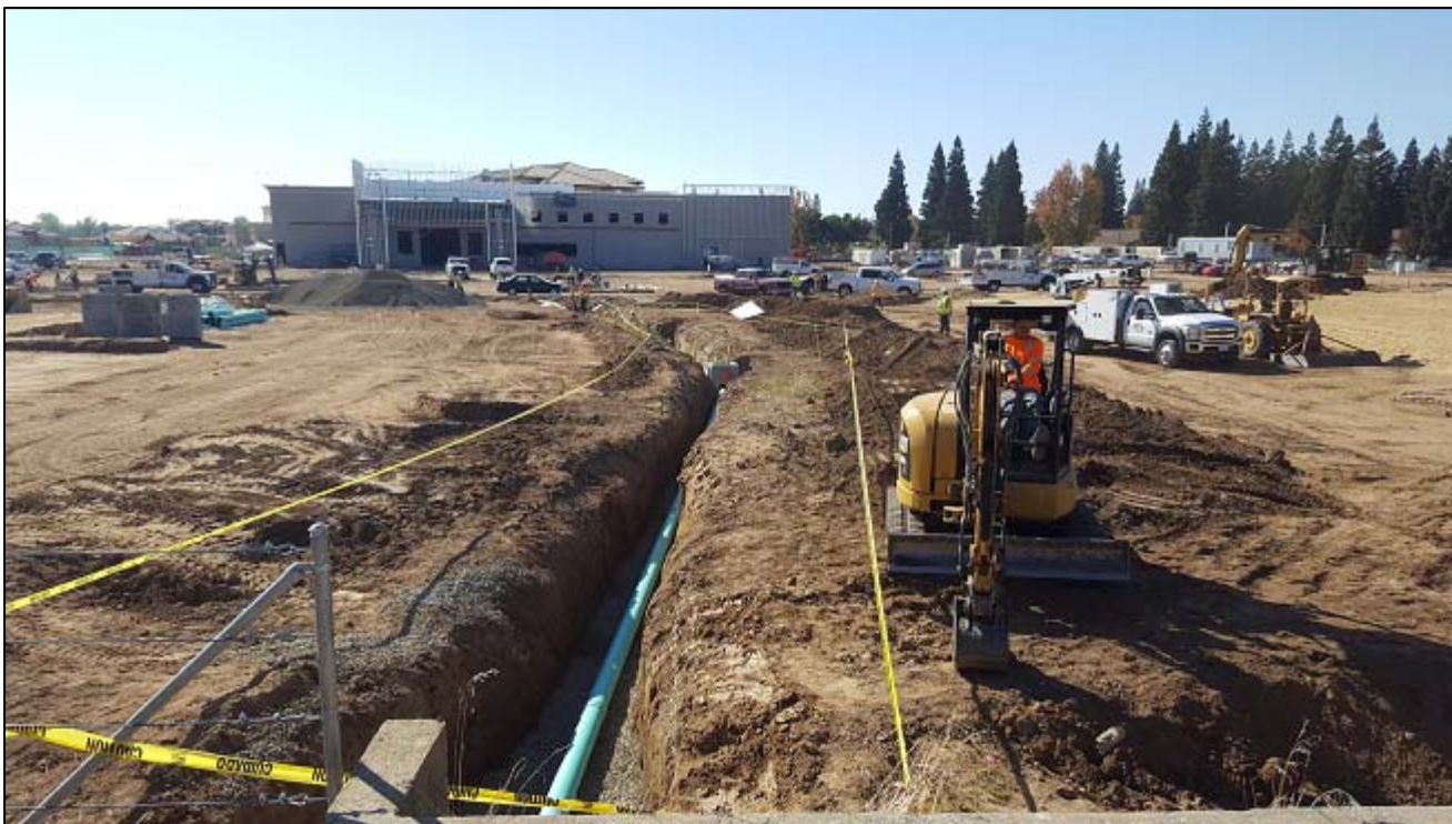
View of storm drain line being installed between lots 4 & 5 with future BelAir in the background
