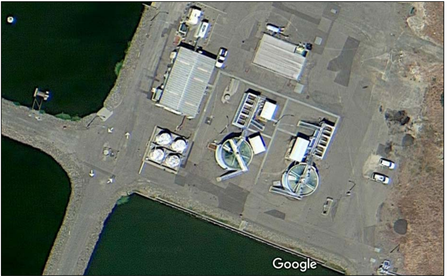
Aerial view of tertiary treatment plant
