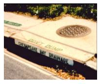
Urban runoff is commonly collected in storm sewers and discharged to waterways untreated, so that any contaminants carried by the storm water are discharged to surface water bodies that are used as the sources of drinking water. In addition, about 20 percent of the population in the U.S. is served by combined sewer systems (for both sanitary waste and storm water) that, during heavy storm events, allow contaminants from sanitary sewage to discharge directly to waterways untreated.
