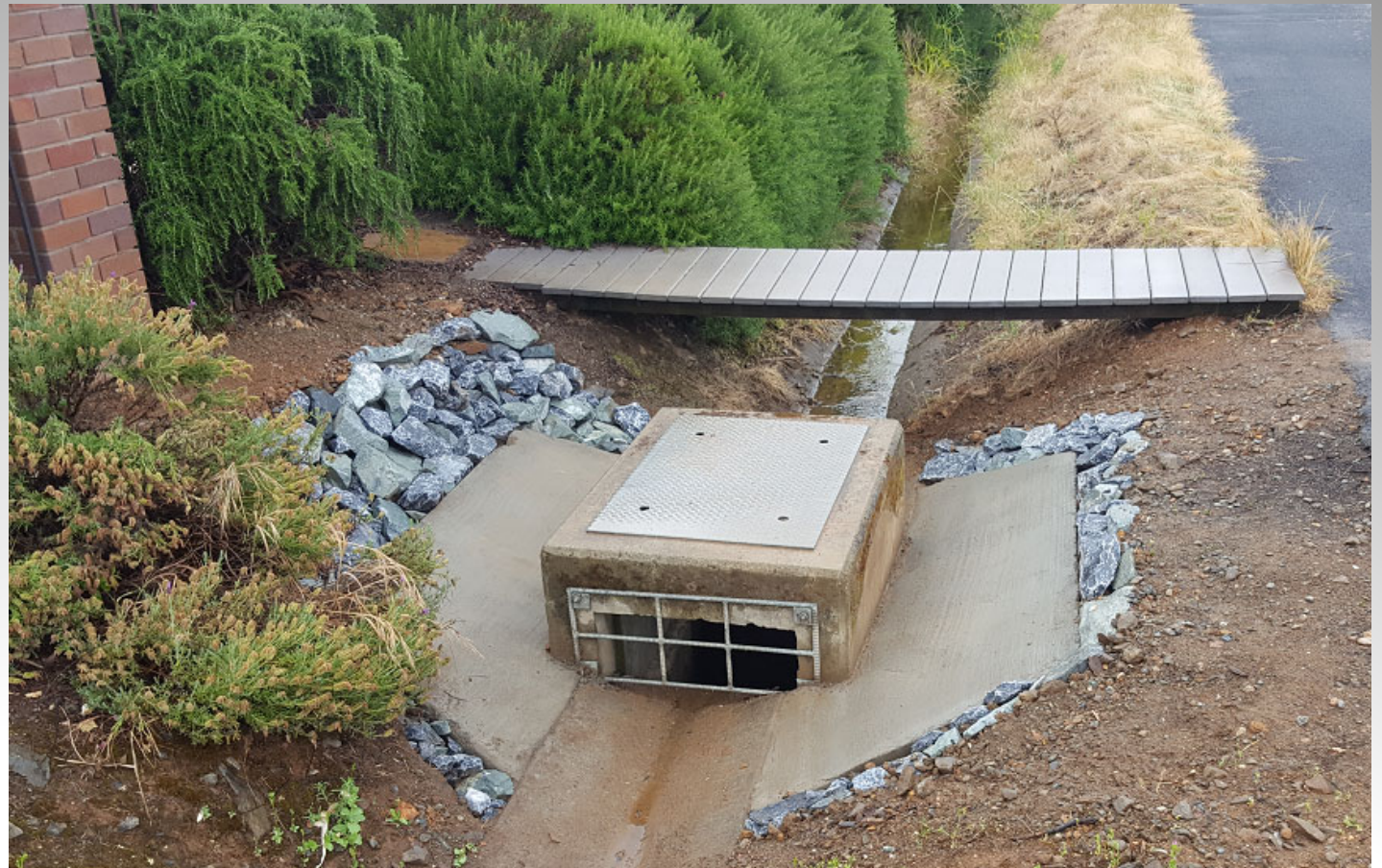
Chesbro drain repair.
