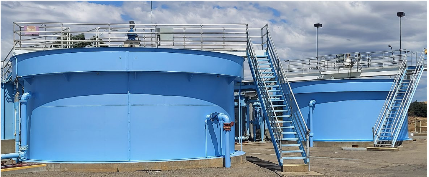
DAF outside paint completed
