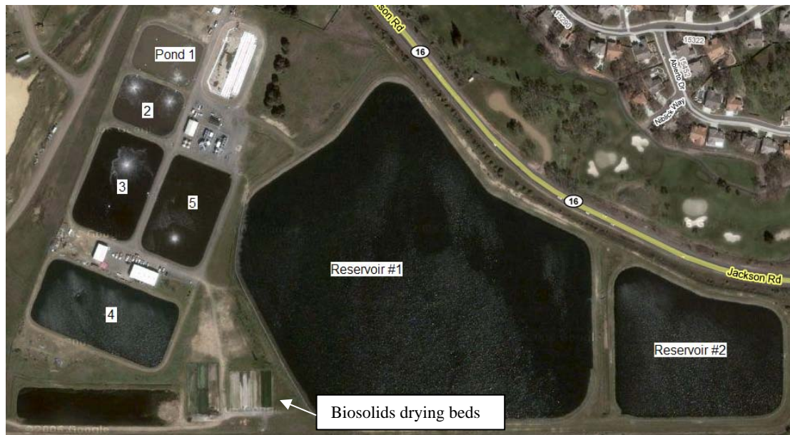
Aerial photo of District Wastewater Treatment Facility
