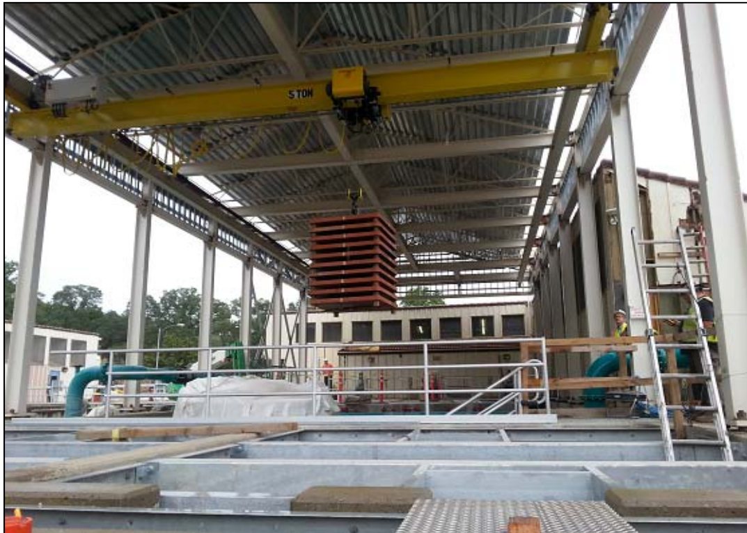
Load testing of crane
