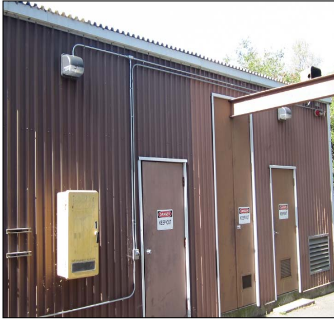
MLN Building showing I-beam and door access for dry well side but none for wet well side
