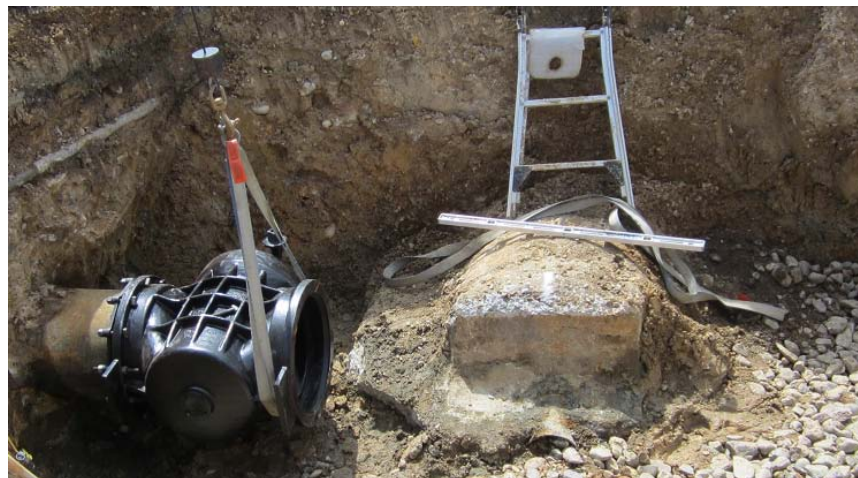
Plug valve being installed.
