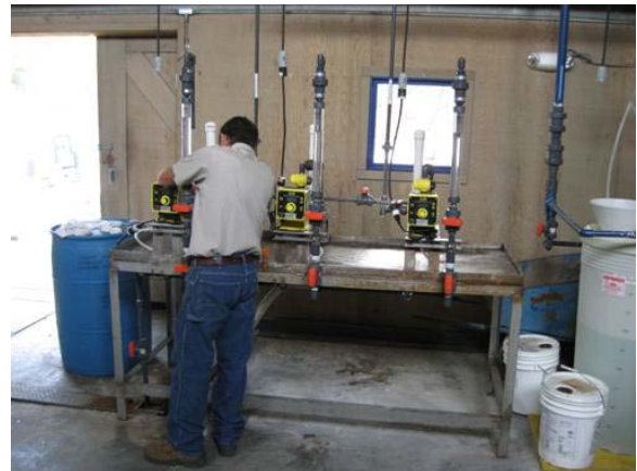
Staff installing new chemical feed lines.
