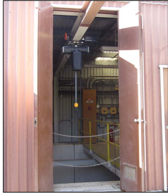
MLN Building showing I-beam and door access for dry well side but none for wet well side
