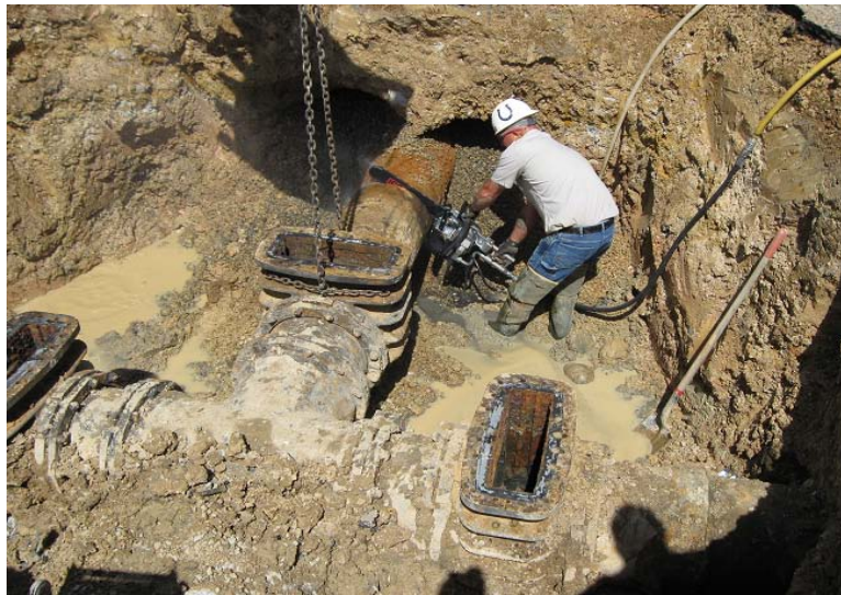
Staff member cutting ductile iron pipe in preparation for valve replacement.
