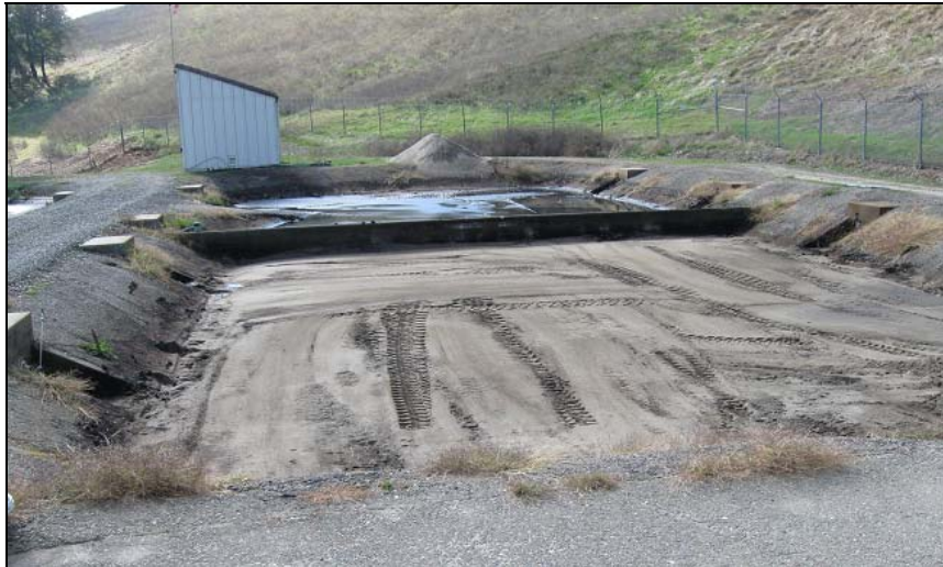
Water Plant solids drying bed after being cleaned out
