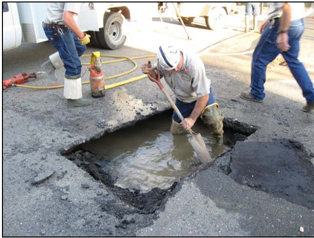
Water line repair on Venado Drive
