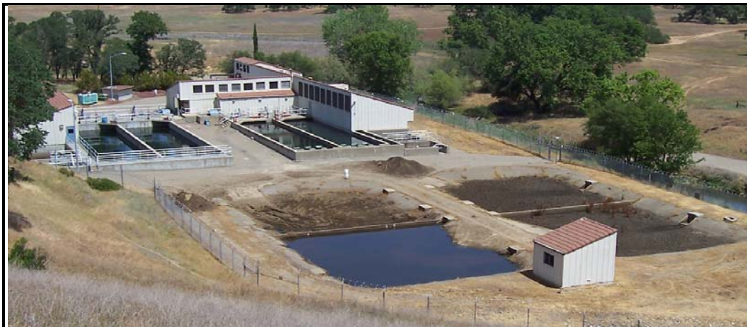
Photo of Water Treatment facility. Plant #1 filter in building on right, Plant #2 filter in building on left.
