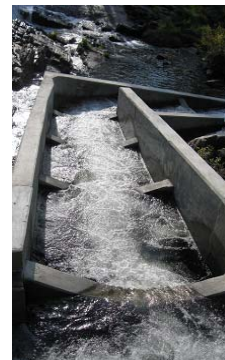
Figure 1 - Granlees North Fish Ladder
