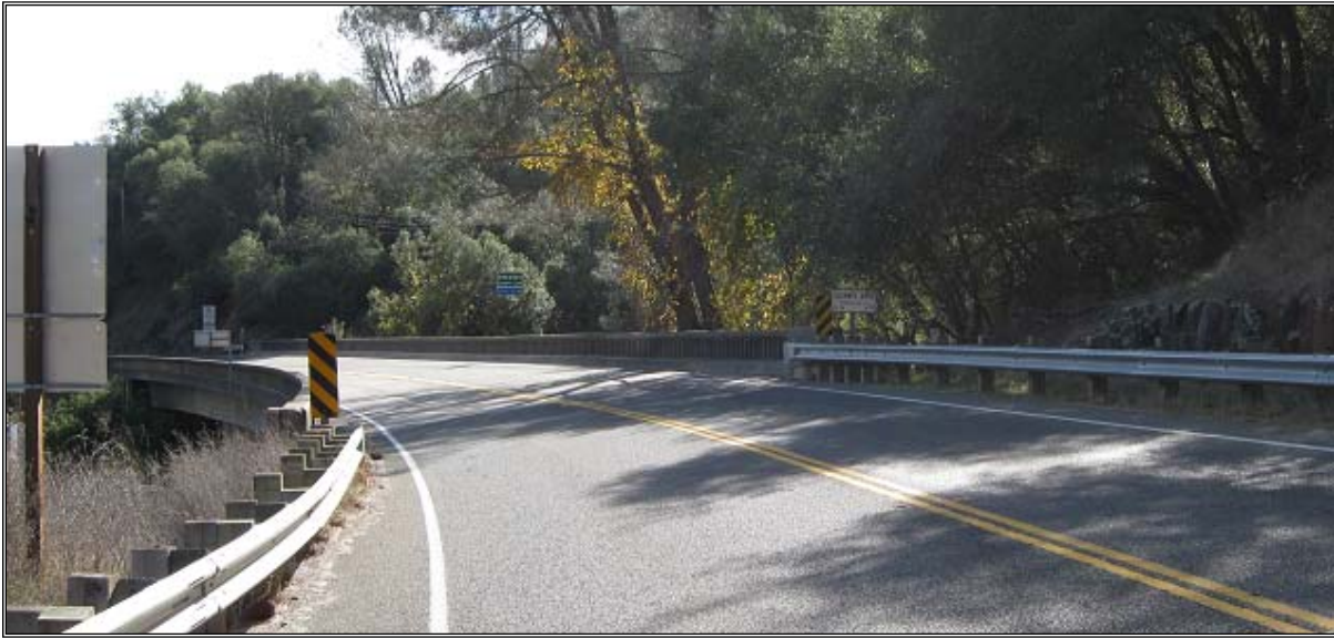
Highway 49 crossing Cosumnes River at Amador & Eldorado county line
