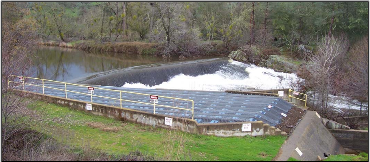
Granlees Diversion structure on North side of Cosumnes River in Rancho Murieta
