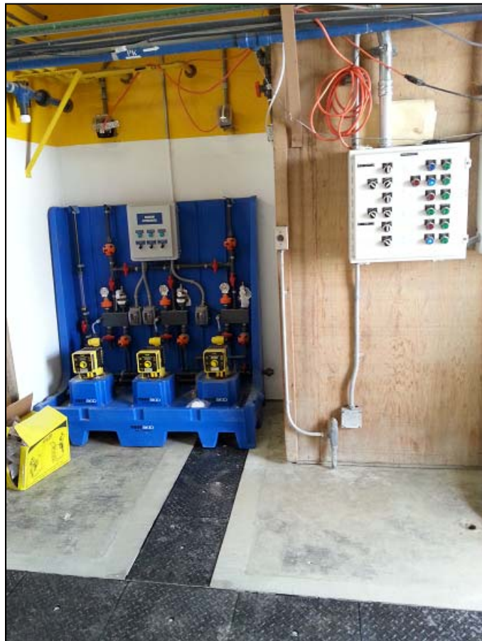
Setting of Sodium Hydroxide Chemical feed skid and new Chemical Trenches
