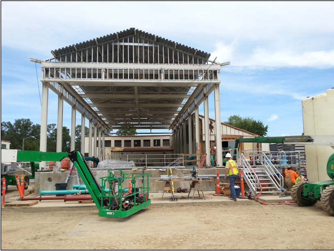
Continuing Erection of Canopy
