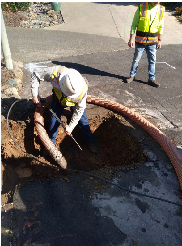
Troy (intern) getting to a water leak
