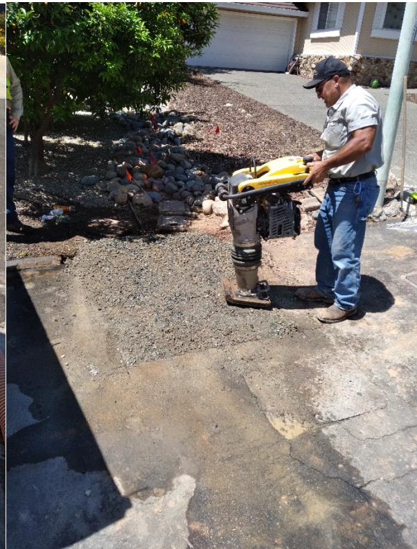
Mario finishing up a water leak
