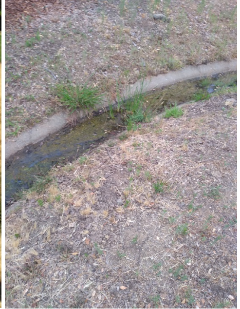
Chesbro protection ditch before cleaning
