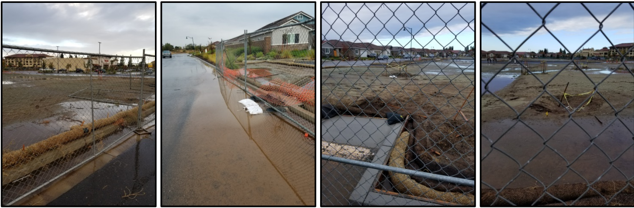
Post Storm pictures
