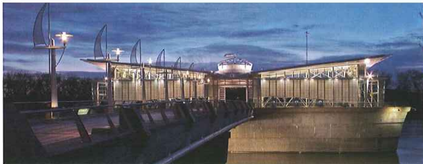
Sacramento River Water Intake Structure, A Tesco Controls project.
