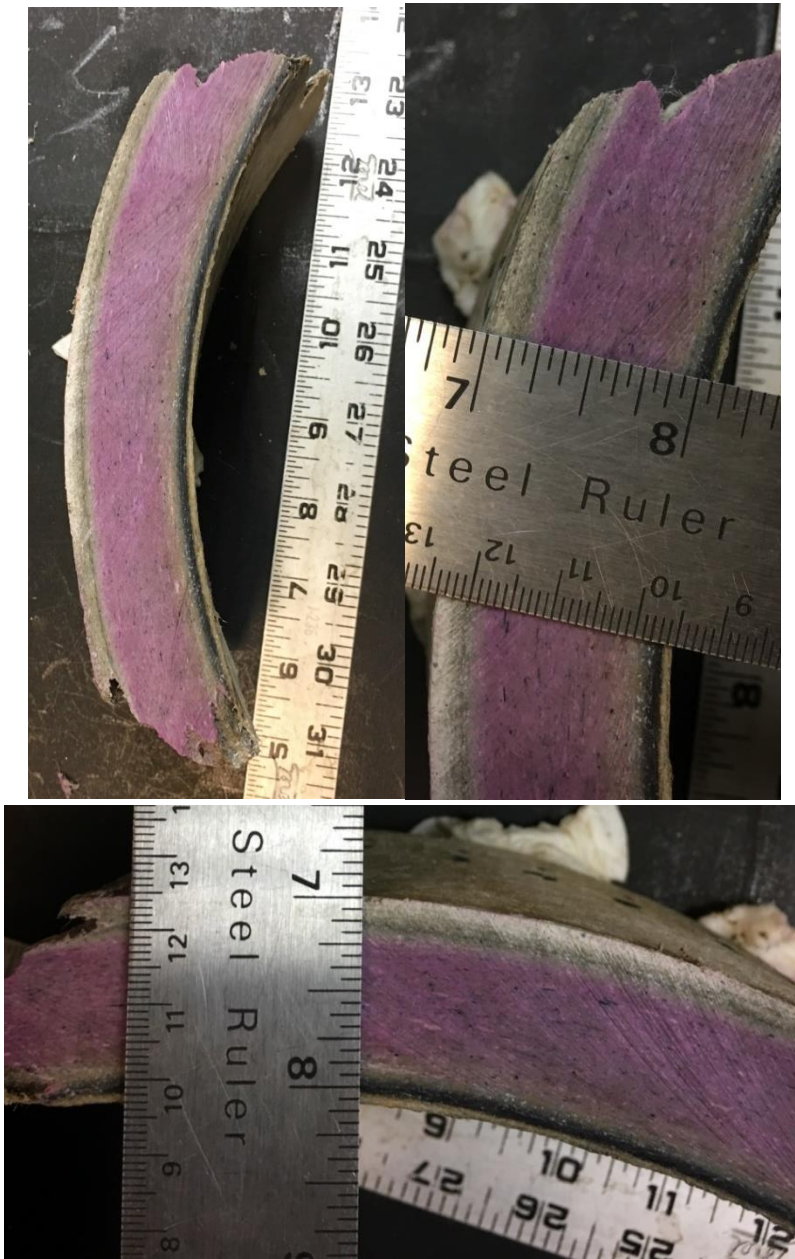
Figure 5: Photographs of Sample 1 wall cross section after staining with phenolphthalein. Note the white areas showing loss of alkalinity
