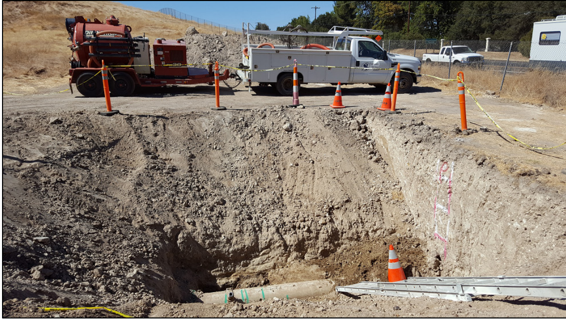
Photo of Stonehouse 12-inch sewer force main pipeline
