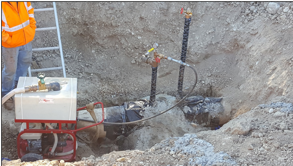
Photo of pressurization of line for integrity test
