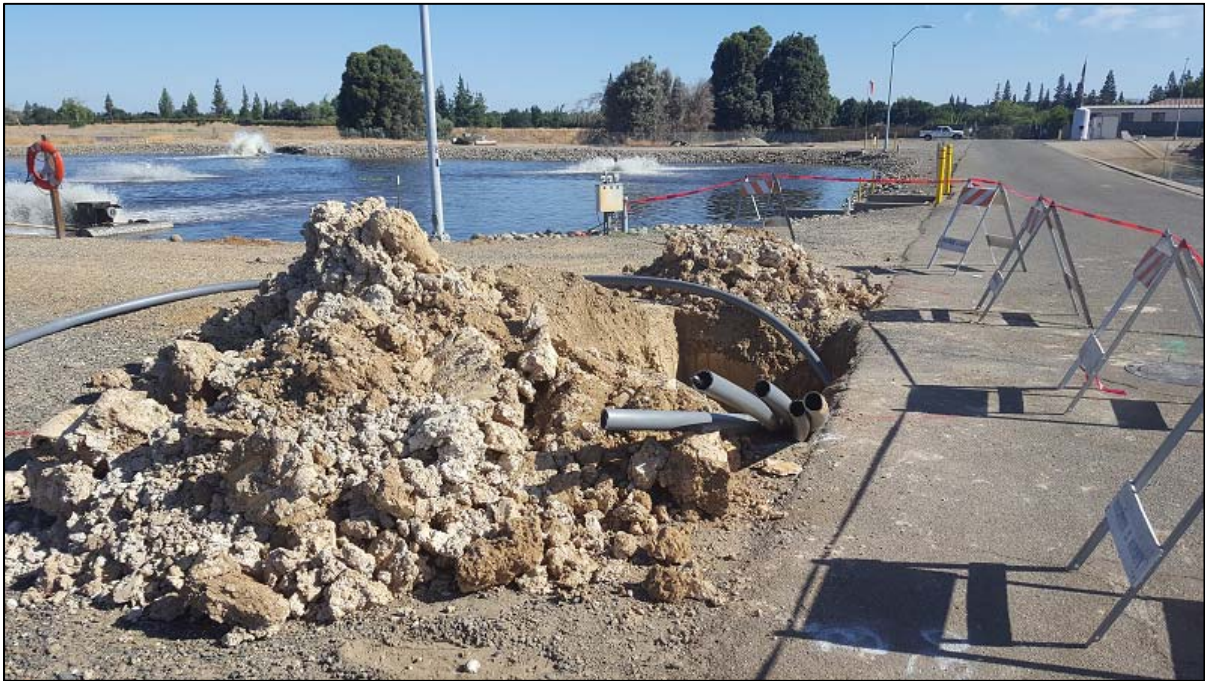
Photo of electrical conduits pulled through bore hole from PV site to Wastewater Plant.
