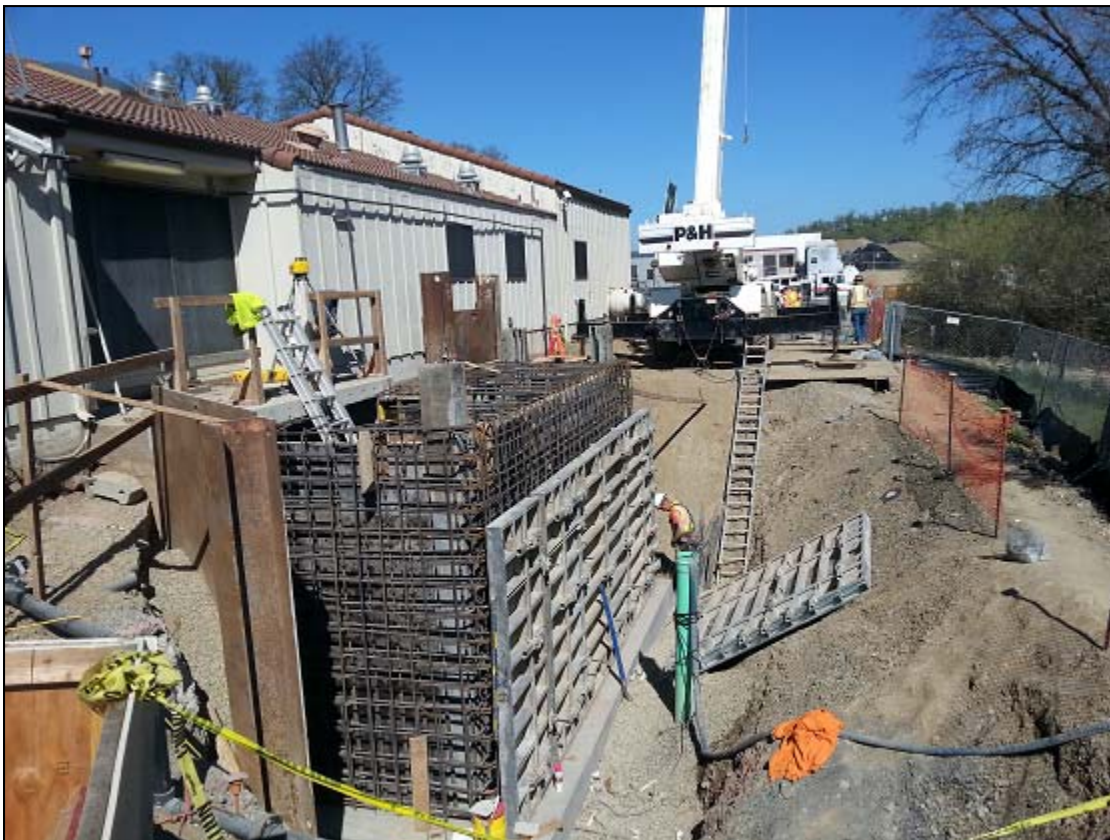
Framing of future effluent discharge pump station
