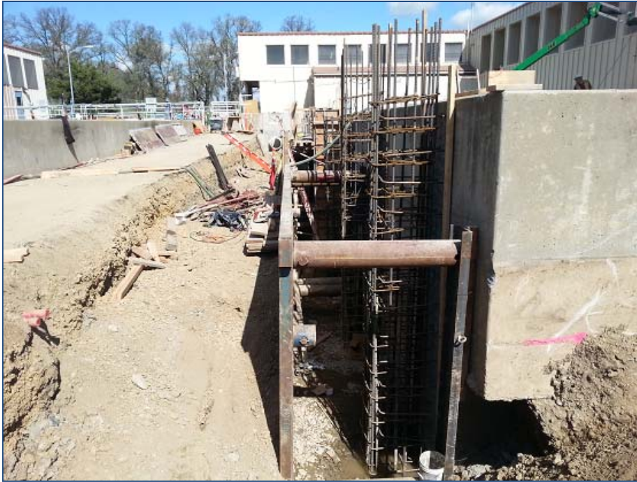
Forming of final pilasters on outside of membrane basins
