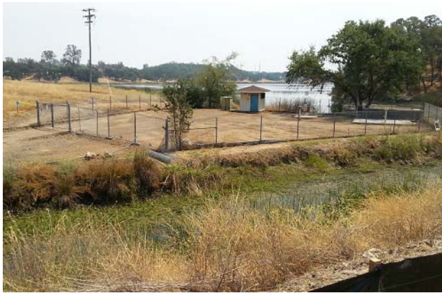
Asphalt grinded off future site of Raw Water Screening System
