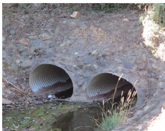
Hole 13N culvert inlet before
