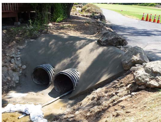
Hole 13N culvert inlet after HDPE pipe installation
