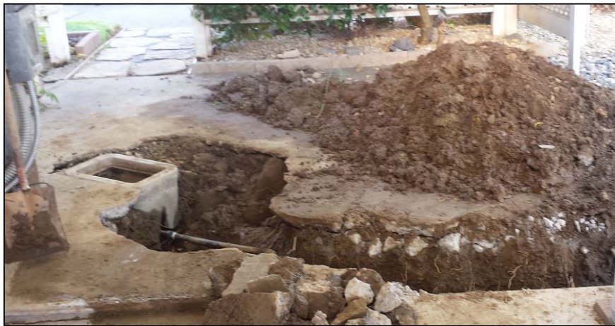
Water service line repair on Golden Circle
