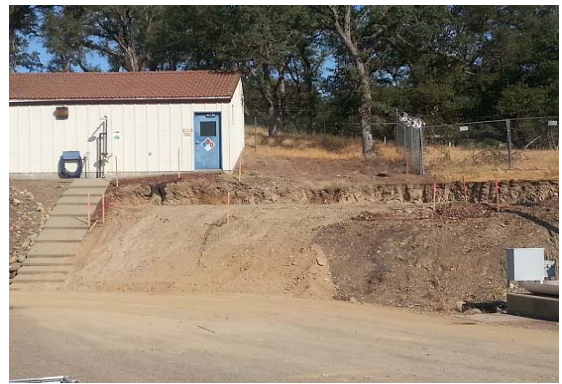
Future site of chemical storage tank installations
