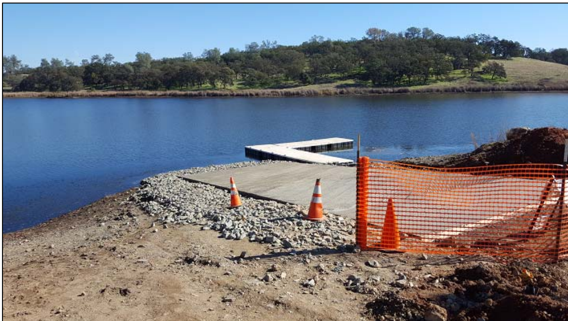
New boat ramp installation at Clementia
