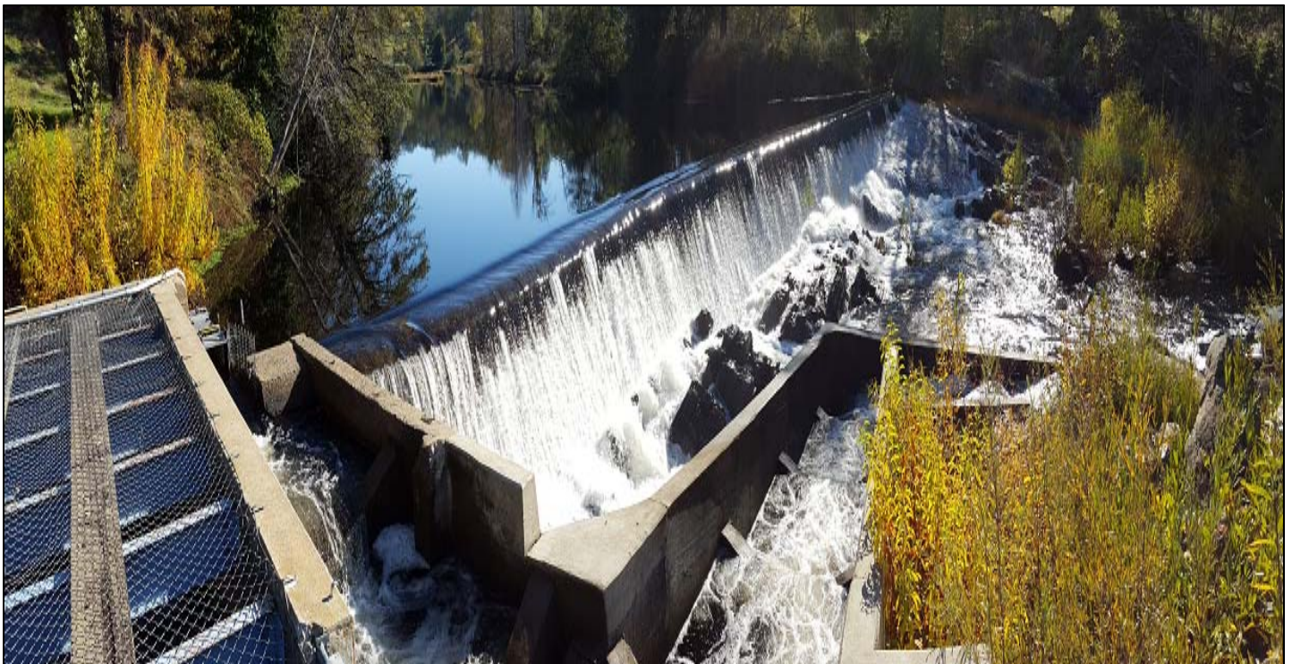
Photo of Granlees Dam with Cosumnes River flow at 232 cubic feet per second.
