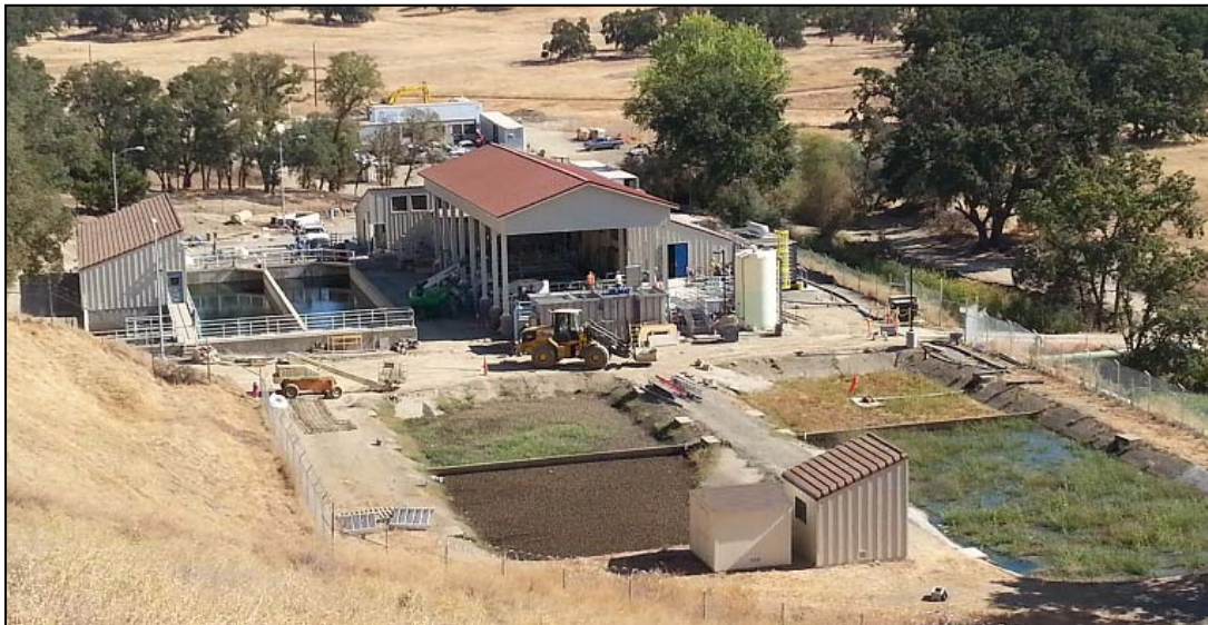
Site overview showing Plant #1 work continuing with Canopy completed.
