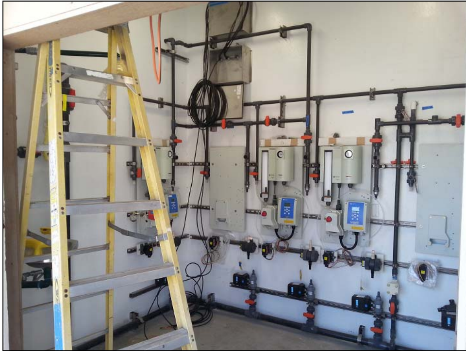
New disinfection control system being installed.
