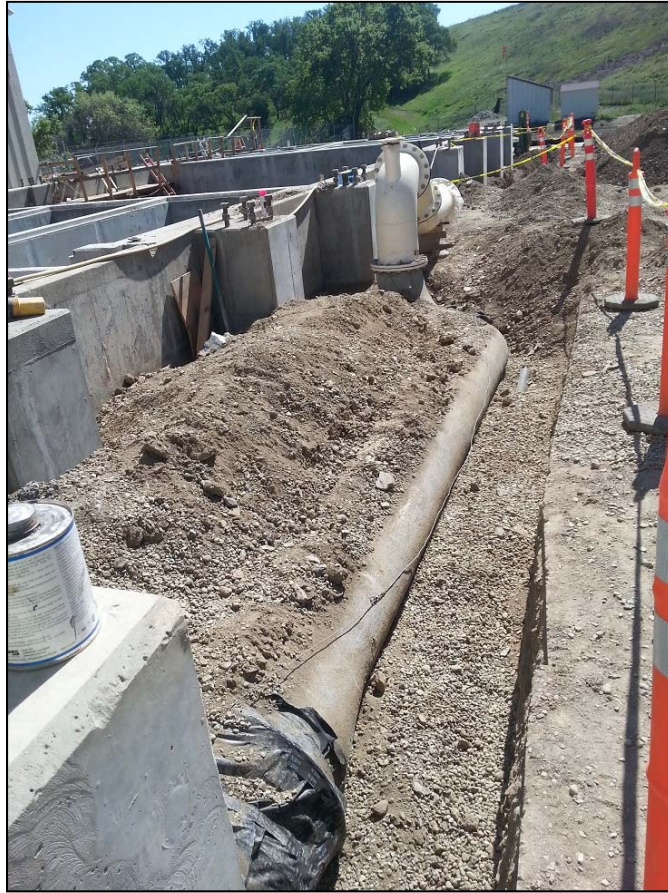
Installation of new 16" Raw Water line
