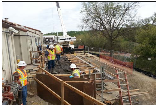
Forming of Effluent Pump station
