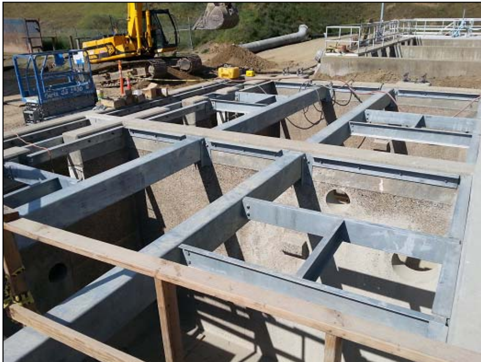
Installation of decking supports on Backwash basins
