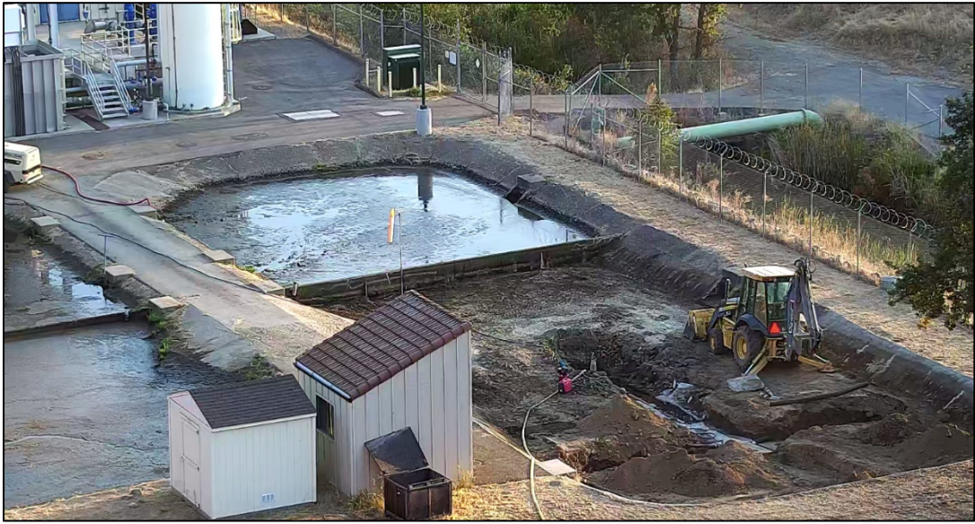
Photo of drying bed piping being excavated
