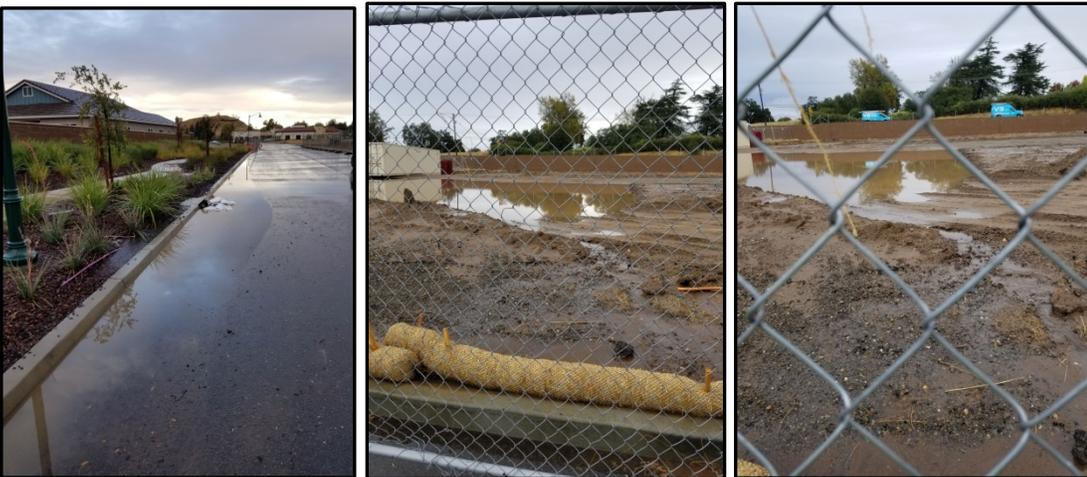
**The Retreats Project.** Project BMPs implemented here are perimeter wattles, street DI perimeter gravel bags, and low point field silt fences. No construction activity has started here yet. If anything some small large concrete pipe quantity has been delivery, and small construction equipment has been stage on site. My observation after the storm on this project has been of no issues all looks good since there is no ground disturbance.
