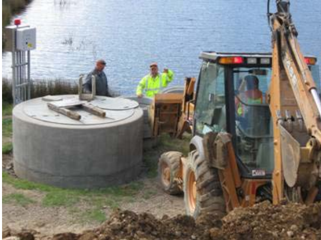
Before and after the backfilling soil around Chesbro siphon vault
