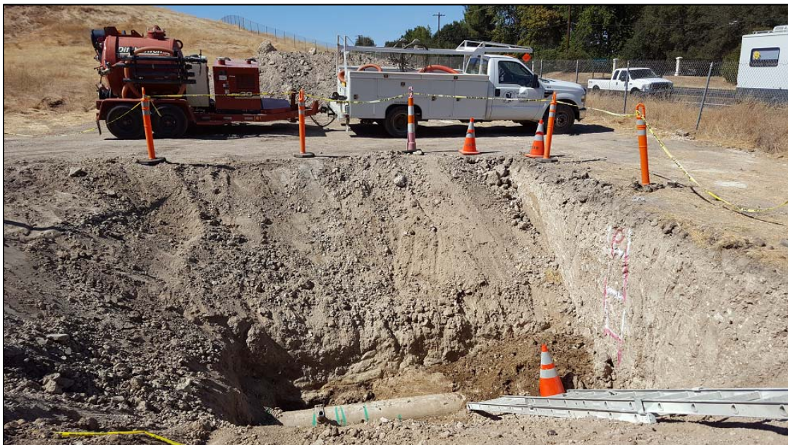
Photo of 12 inch force main pipeline to possibly be used for future conveyance of recycled water.
