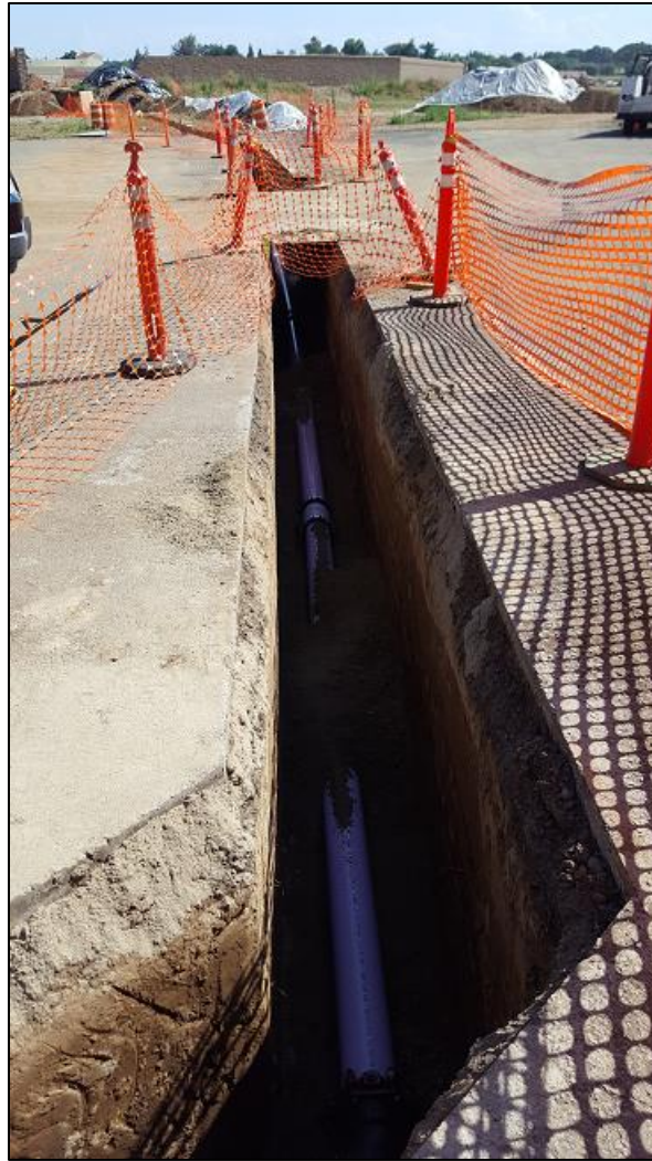
Newly installed 6-inch recycled water line.
