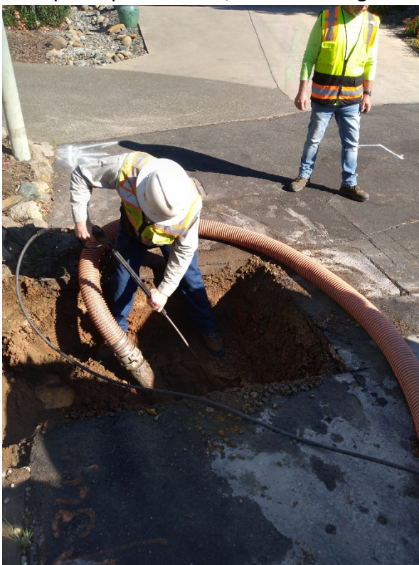
Troy (intern) getting to a water leak
