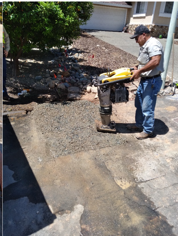
Mario finishing up a water leak
