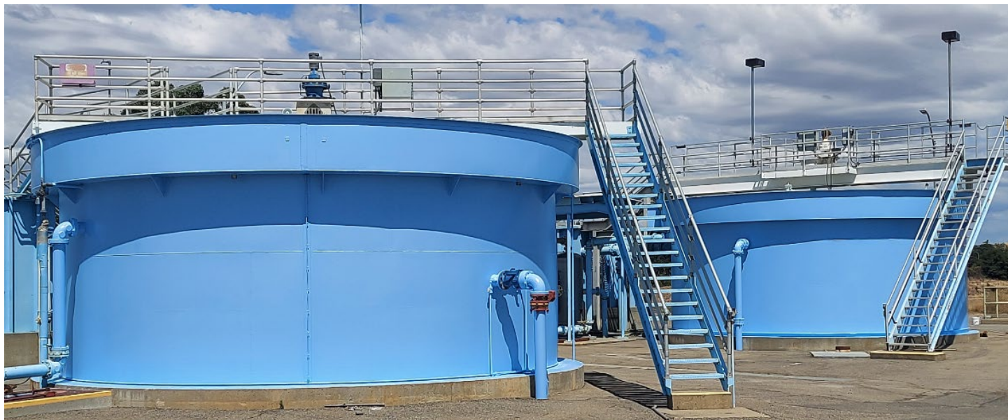
DAF outside paint completed
