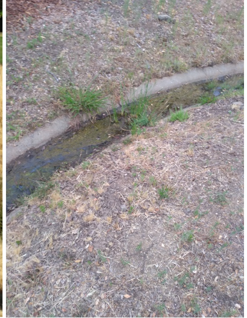
Chesbro protection ditch before cleaning
