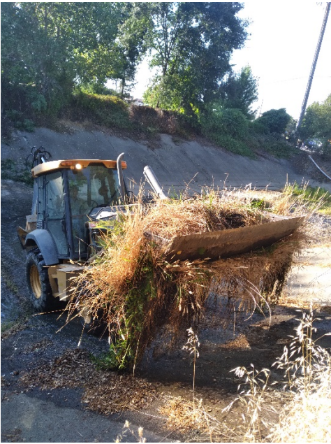
Cleaning Debris from Laguna Joaquin spill way
