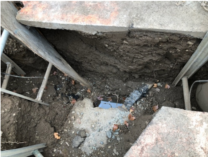
Photo 2: Trench excavation after initial backfill dated 12/13/18. Concrete area in middle of trench is top of thrust block on existing 90 degree bend.
