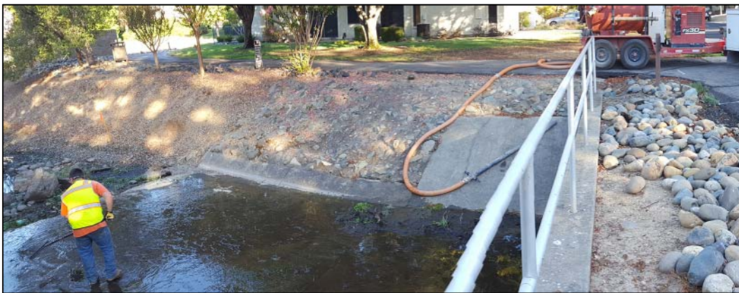
Photo of Utility staff cleaning up inlet to Laguna Joaquin
