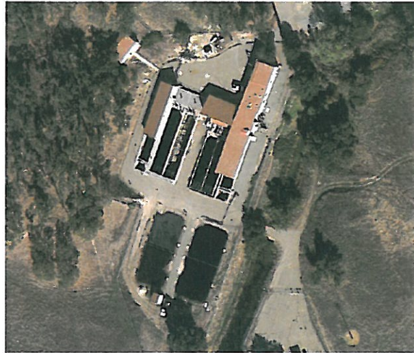
Figure 3 RMCSO WTP #1 (right) and #2 (left)
