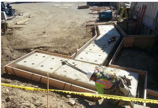
Chemical trench vault installation
