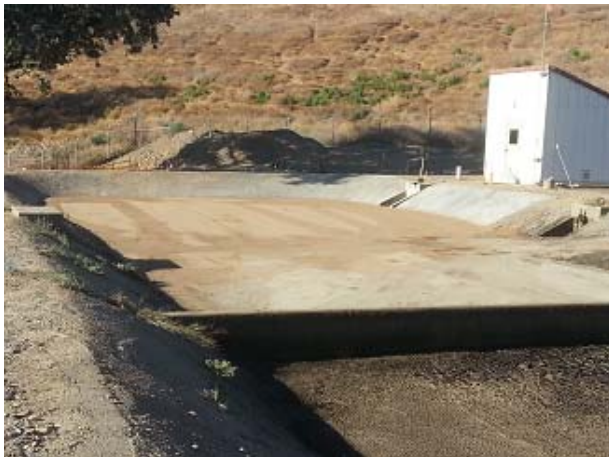
Drying bed extension completed
