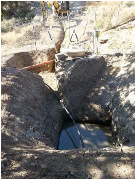
Sewer force main installation from Water Plant to Clementia Circle
