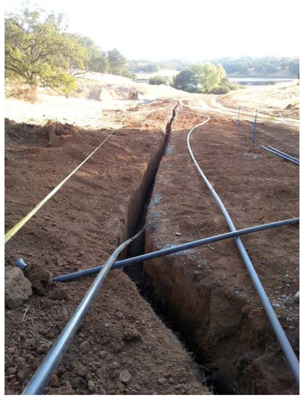
Photo of new sewer line extension
