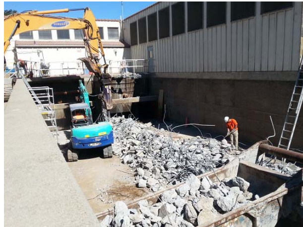
Demolition of sedimentation basins
