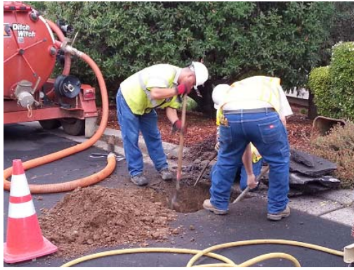
Utility staff making water line repairs on Robles Grandes and Camino Del Lago
