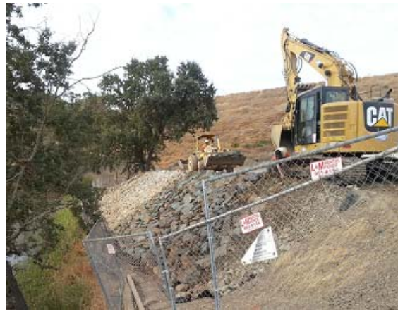
Embankment protection below drying beds
