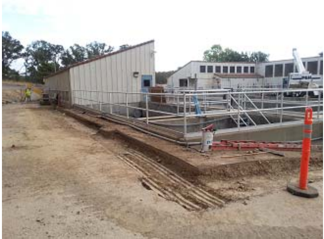
Twelve inch (12") Filtrate line install around Plant #2
