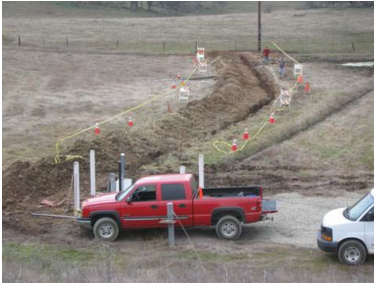
Trenching to run new power supply to Calero's East Dam Subdrain
