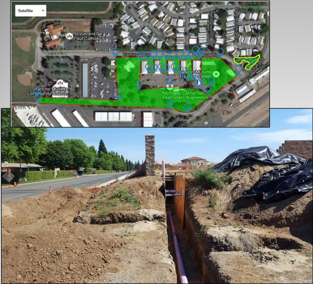
Photos of 6 inch recycled water line running towards Cantova Drive from Murieta Gardens Lot 66
