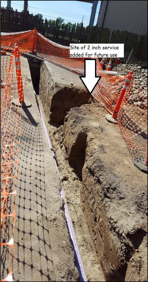
Photos of 6 inch recycled water line running towards Cantova Drive from Murieta Gardens Lot 66
