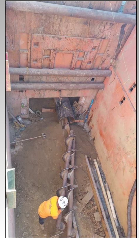
Photo of point of connection from recycled water line going to Bass lake to Murieta Gardens/Commercial areas Boring under Highway 16
