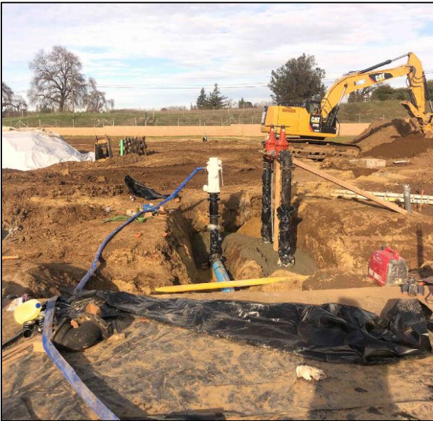
Fire hydrant installation on Lot 5 of Murieta Marketplace project
