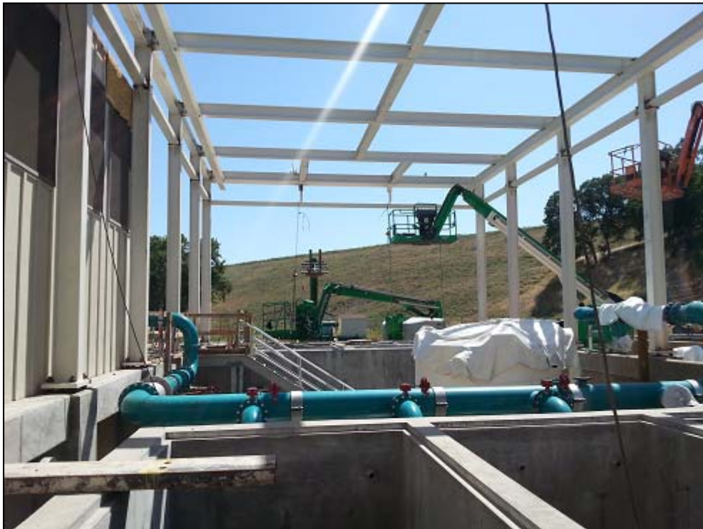
Canopy Structure framing nearly completed
