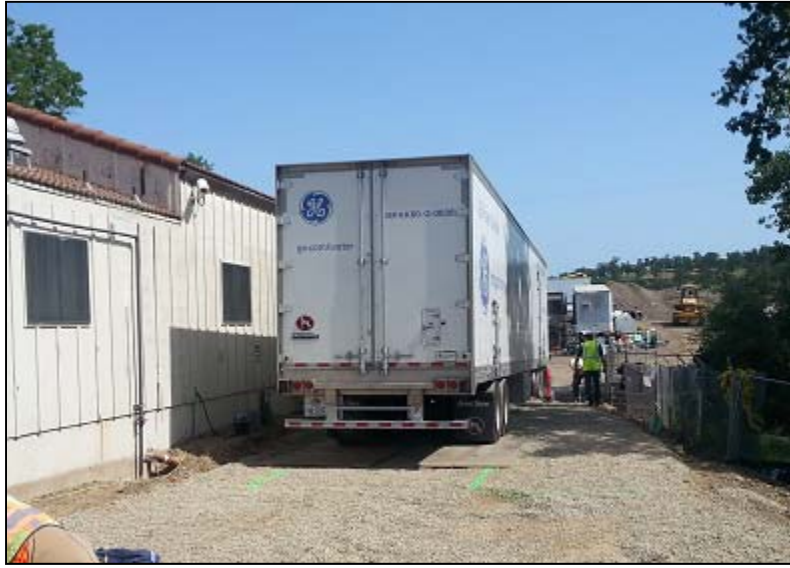
Temporary Filtration System being set in place
