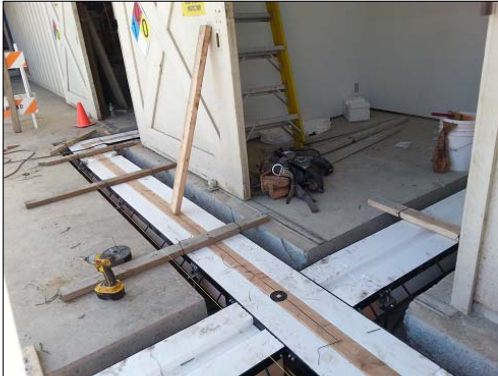
Membrane permeate pumps and beginning of piping installations
