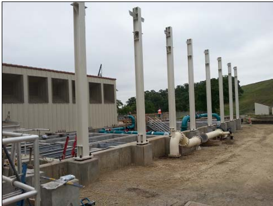
Erection of Canopy structure
