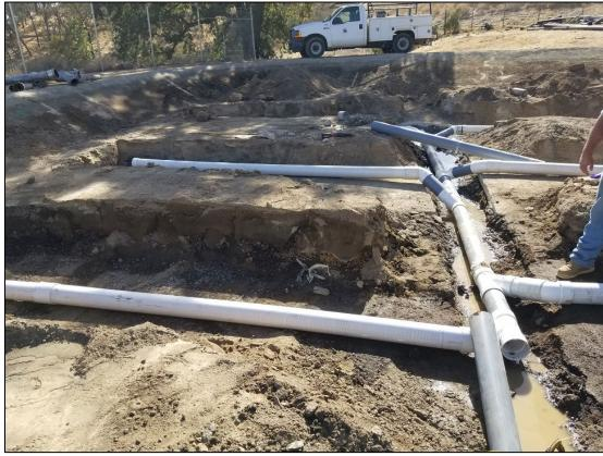
Photo of general layout of pipes before direction of sweeps were corrected
