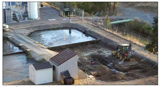
Photo of drying bed piping being excavated
