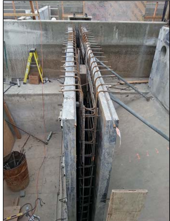
Forming of future back-pulse basin wall.
