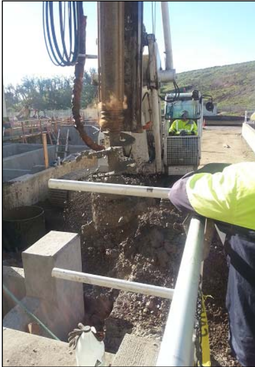
Drilling for pilasters on outside of membrane basins.
