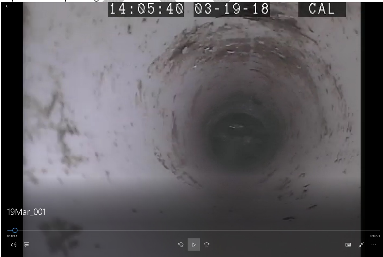
Capture #2: Scope being lowered down shaft of cleanout
