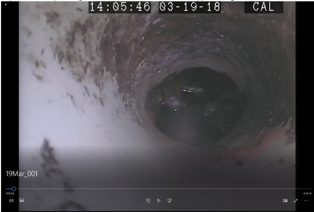
Capture #3: Scope being lowered down shaft of cleanout approaching cleanout "Y"
