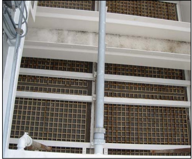
Wastewater Plant filter cell with sand removed showing screening.
