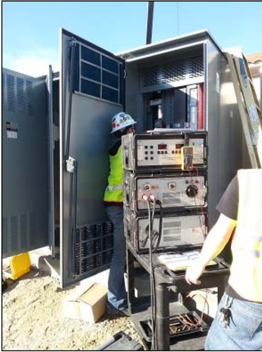
Testing of electrical switchgear installation.
