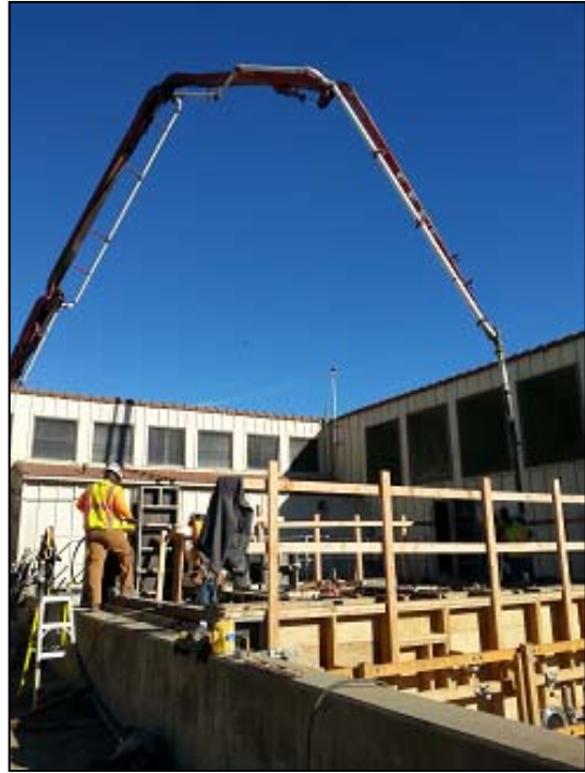
Pouring concrete for membrane basins.
