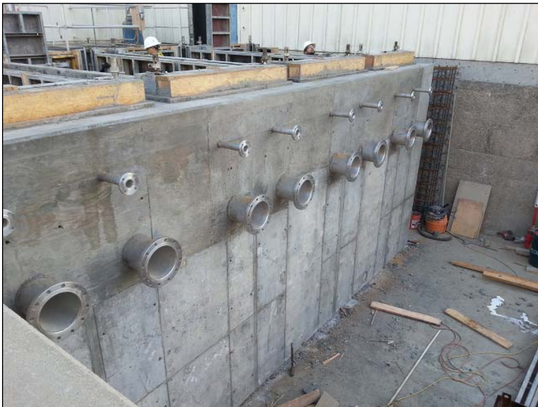
Discharge side of future membrane basins after concrete forms removed.
