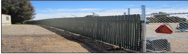
Newly installed security fence along Wastewater Reclamation Facility
