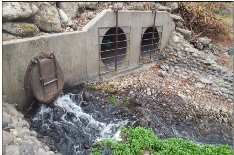
Basin 5 river outfall and Main Lift South Storm pump outfall
