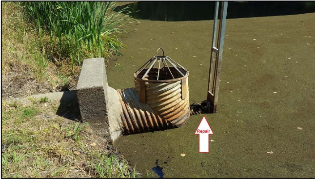
Photo of low flow outlet before and after repair at Basin 5
