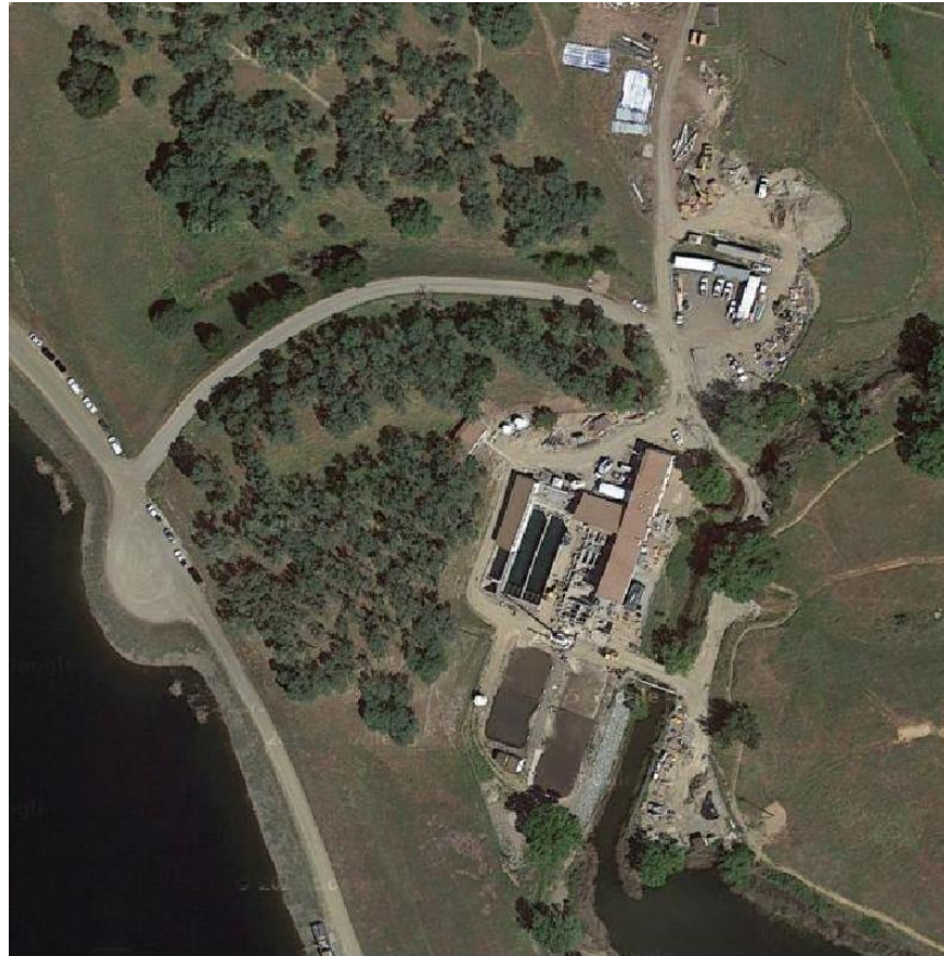
Aerial overview during construction
