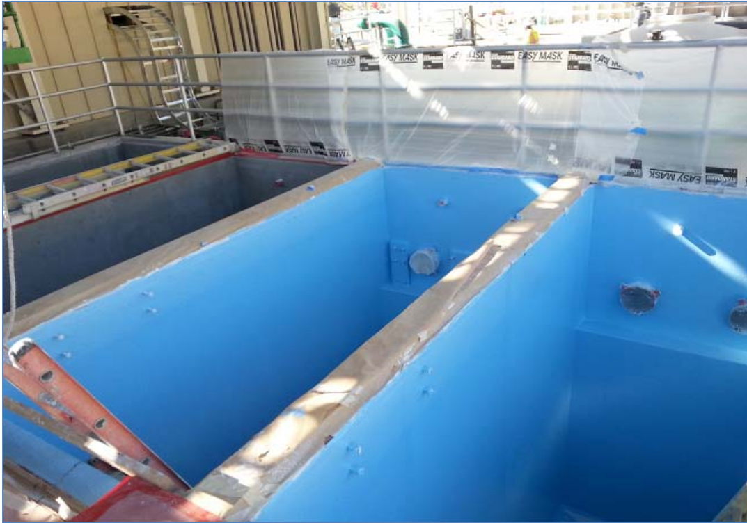
Coating of membrane basins
