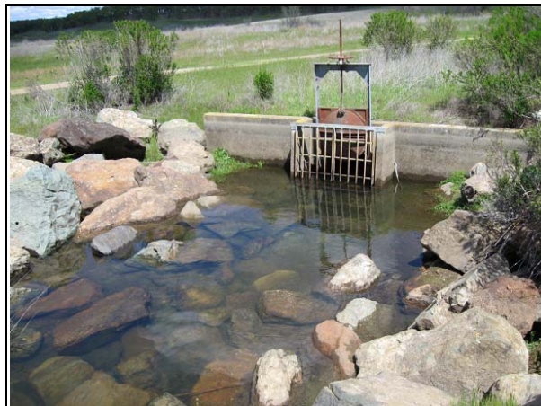
Inflow structure at Calero Reservoir on April 5, 2012.
