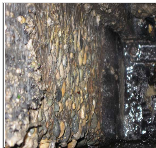
Photos showing exposed aggregate due to corrosion of concrete in Main Lift North wet well #1 & #2
