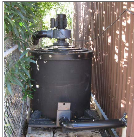
Sewer gas "Air Scrubbing" system installed to vent and neutralize sewer gases from the wet wells.
