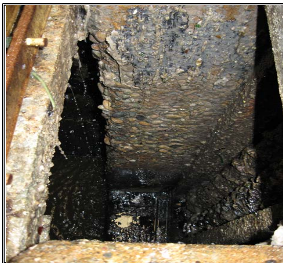
Photos showing exposed aggregate due to corrosion of concrete in Main Lift North wet well #1 & #2
