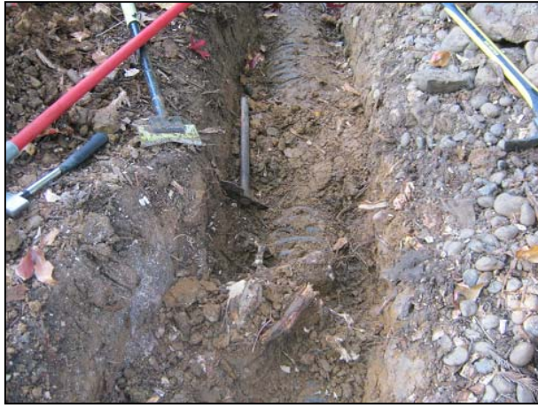
Unapproved Drainage line discovered with roots in it, removed by staff.
