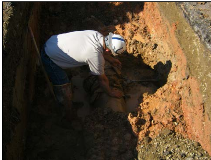
Staff repairing a leaking service line on Murieta South Parkway.
