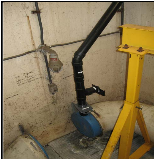
Sewer gas "Air Scrubbing" system installed to vent and neutralize sewer gases from the wet wells.
