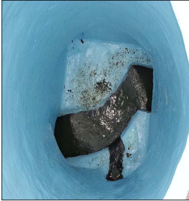
Photos of completed rehabilitation of manholes that feed the Main Lift North sewer pumping station
