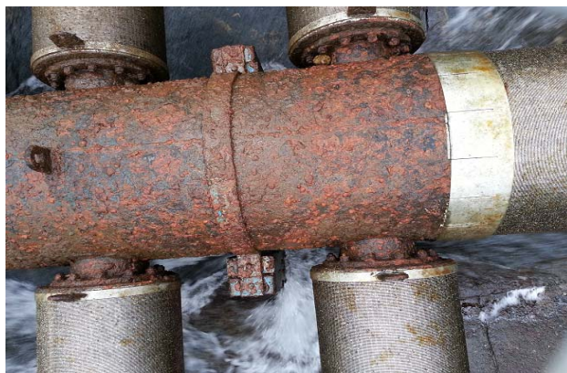
What the intake screens look like, consisting of a fine stainless steel mesh
