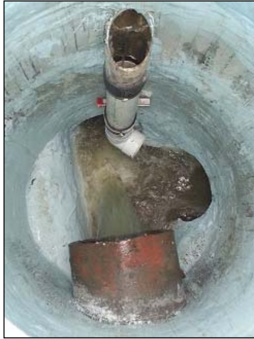
Photos of completed rehabilitation of manholes that feed the Main Lift North sewer pumping station
